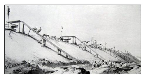
The navies were on 'piece work' so needed no prompting to move a goodly tonnage of spoil. Of course, with such a long high cutting adequate drainage from the cutting was needed and below track drains.
